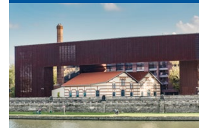
Municipal Power Station, photo by Joanna Górlach
